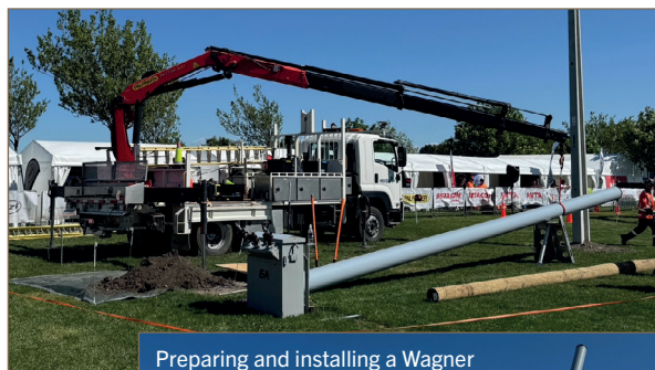
Preparing and installing a Wagner composite pole under the watchful eyes of the NZI exhibit stand.
